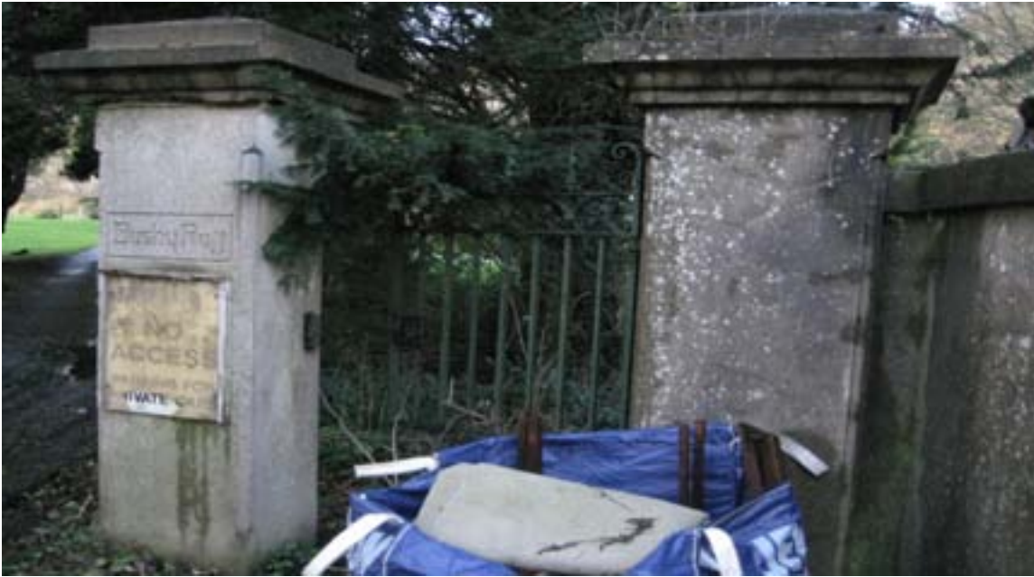
Figure 18. Entrance posts and railings
