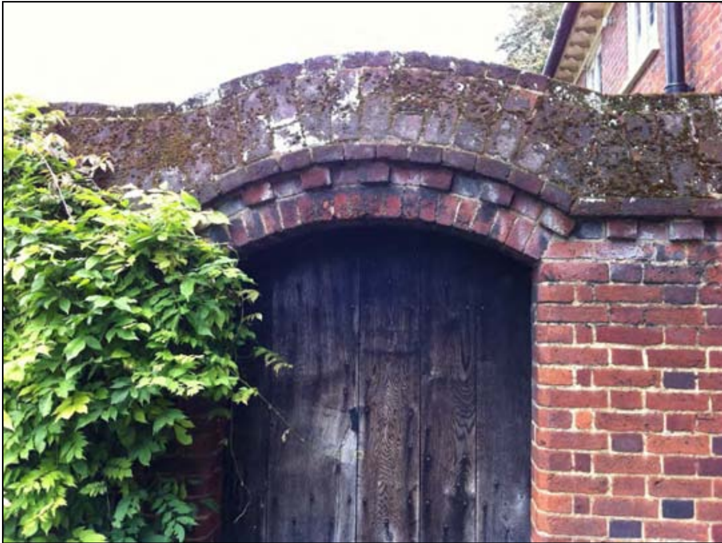
Fig. 21 The Dawber arched-doorway showing dentilled and Flemish-bond brickwork. September 2013
