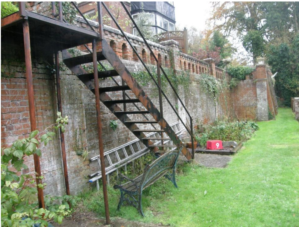
Figure 23. Metal staircase to give access to garden 2014
