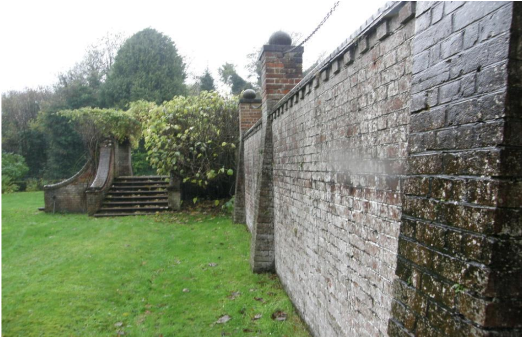
Figure 19. Terrace Walls & Steps 2014
