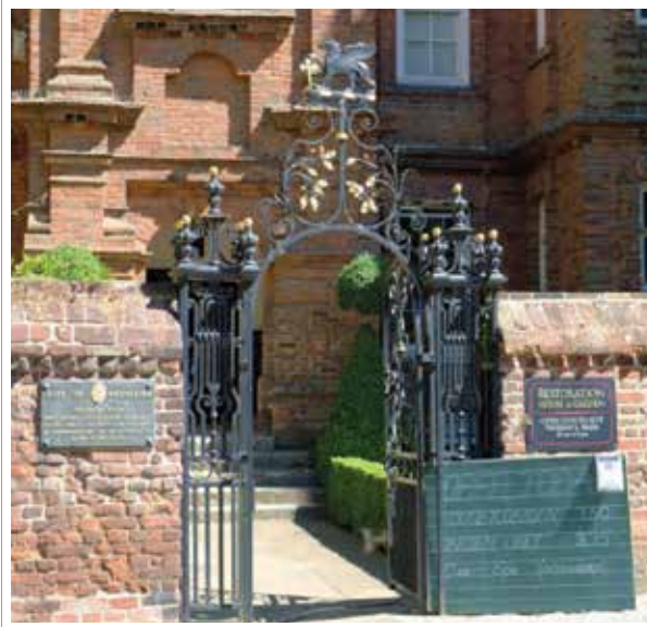
The Entrance gates
